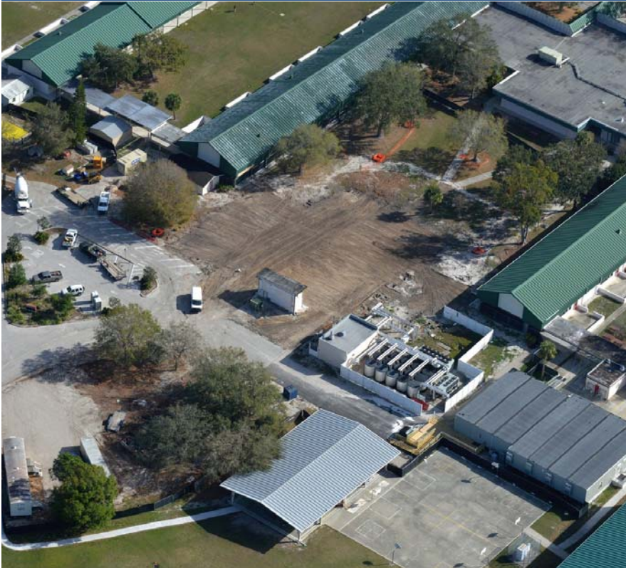
Photo 1: Aerial of Demolished Cafeteria and Temporary Cafeteria
