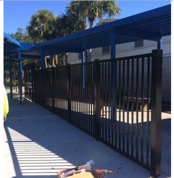
Photo 2: New security fencing being installed
