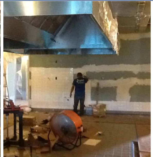
Photo 2: Wall tile being installed in Culinary Kitchen.
