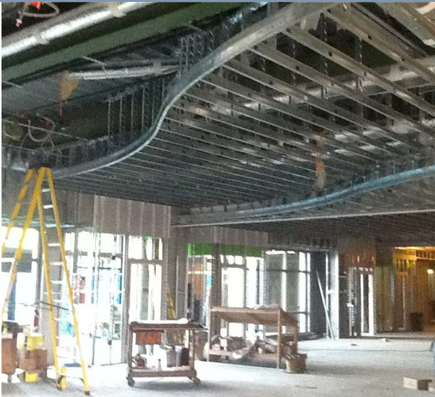
Photo 1: Framing at curved drywall soffit in Conference Center.
