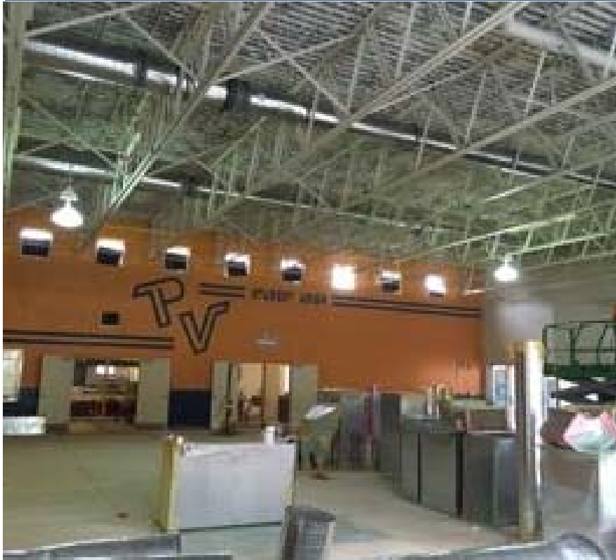
Photo 1: Ductwork ready to be installed in Student Union.
