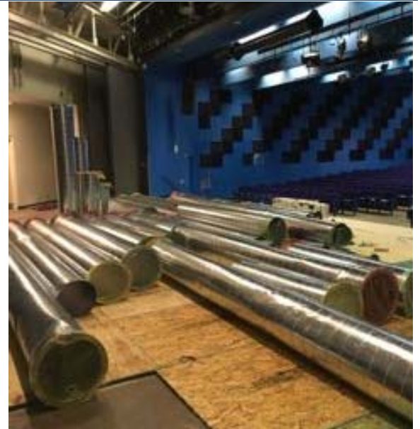
Photo 2: Ductwork ready for installation in Auditorium.
