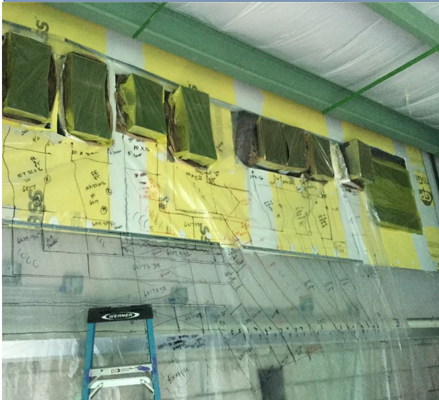
Photo 1: Ductwork coming through wall into bump-out ready for final tie-in.
