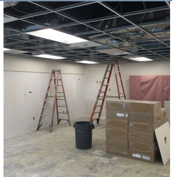
Photo 2: New ceiling grid and lighting installation.
