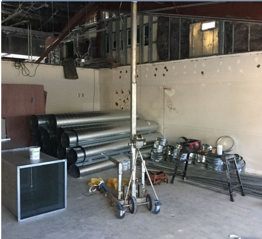
Photo 1: Ductwork ready for installation.
